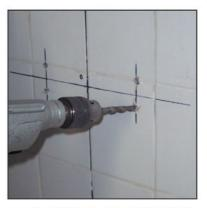
Place the (+) sign on the adjustment with the intersection point, mark the holes of the mounts on both sides. Drill the marked points with suitable bits and insert raw plugs.
