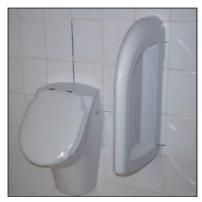
Test the urinal for any leakage. Protect the item until the end of construction works.
