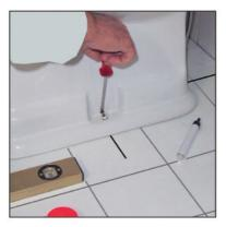
Place the bidet to its final position and fix it by using its original assembly kit.
