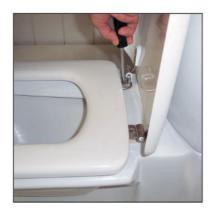
16 Use a simple cross-head screwdriver to tighten the seat cover.
