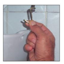
9 The hook of the assembly kit is fixed on to the hole of the semi pedestal.
