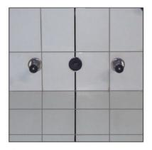
1 The waste water centre (Ø50 mm) is prepared at 125 mm above the finished floor. Set the gap between interval tap inlets to 400 mm. symmetrically regarding the centre as basis.
