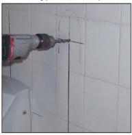
Draw vertical axis for wall seperator assembly parts, as shown on product pages. Drill the intersection points with 10mm. bit, insert raw plugs.
