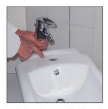
Set the gap between interval tap inlets to 400 mm. symmetrically regarding the centre as basis. Install the tap.
