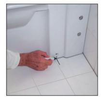
Use the projection of the WC pan and assembly holes at sides as template and trace contour lines on the floor.
