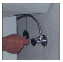
After fixing the washbasin, make the connections between interval taps and basin tap with 3/8" flexible connection pipe.
