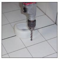
Drill the marked points with suitable drill bits and insert the raw plugs.
