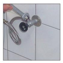
11 Check the final balance with a water gauge. Test the bidet and interval taps for a possible leakage. Silicone based pastes may be applied on the joining edges of the ceramic and finished wall for a better tightness and aesthetic view.
