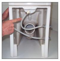
13 Check all connections and hoses against leakage.
