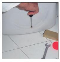
Place the wc pan to its final position and fix it by using its original assembly kit.
