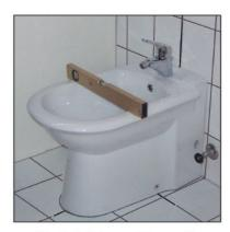
Place the bidet temporarily to assembly position. Use the assembly holes as reference points and mark the projections on the finished floor.
