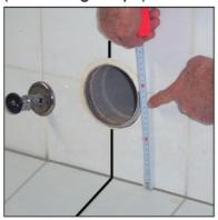
The centre of waste water outlet on the wall must be set to 170 mm. above the finished floor and the same level with the finished wall.
