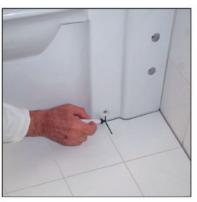
5 Use the projection of the WC pan and assembly holes at sides as template and trace contour lines on the floor.
