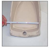
3 Check out the gap between two edges behind the urinal.
