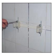
6 Fix the stick with assembly mounts on it.
