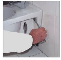
Push the bidet forward to assembly position. Slide the syphon trough the waste water outlet. Fix the assembly nuts of the bidet.
