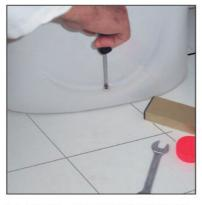
Place the wc pan to its final position and fix it by using its original assembly kit.
