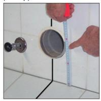
Set the distance between the outlet of the wo pan and the finished floor. Consider the slope required for the flow of the waste. Prepare the waste water outlet on the wall.
