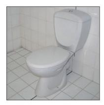
Test the wc pan for a possible leakage. Silicone based pastes may be applied on the joining edges of the ceramic and finished wall for a better tightness and aesthetic view.
