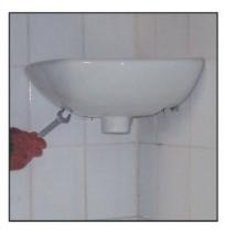
Mount the tap and syphon on the corner basin. Place the basin on the assembly bolts, insert the plastic bushes and fix the bolts with nuts.
