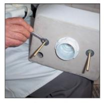
3 Install the flushing mechanisms to the cistern.
