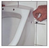
Place the urinal temporarily to assembly position, mark the projection of the product and assembly holes intersect vertical and horizontal axis.
