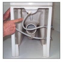
12 Check all connections and hoses against leakage.
