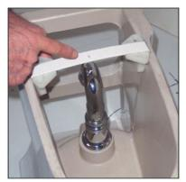
Place the main mounts on the strip. Check the gap now with strip; mounts on it. The length of the strip may neither long nor
