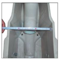
For a proper assembly; check the gap at the foot of the WC pan. NOTICE: This dimension may vary upon each item. So, check each WC pan individually before commencing the installation.
