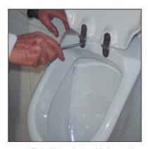
12 Fix the lid by using its original assembly kit.
