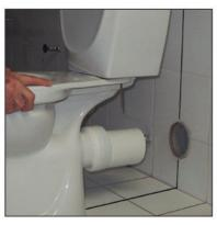
Slide the eccentrical trap adapter to the outlet of the wc pan. Calculate the gap, which is needed for extension for the waste piping.
