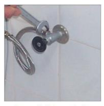
4 Prepare and finish the connections between bidet tap and interval taps.
