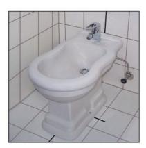
Check the final balance with a water gauge. Test the bidet and interval taps for a possible leakage. Silicone based pastes may be applied on the joining edges of the ceramic and finished wall for a better tightness and aesthetic view.
