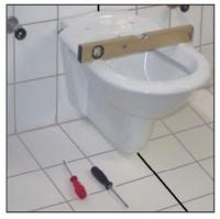
Place the wc pan to final assembly position and fix it by tighten the nuts trough the assembly bolts of the recessed cistern.
