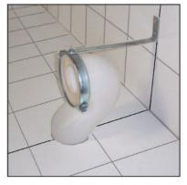
Fix the special "S" pipe to the ring, join the "S" pipe with the waste water pipe on the floor. Fix the ring to the wall with "S" pipe on it
