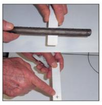
For a proper assembly; check the gap at the foot of the bidet. NOTICE: This dimension may vary upon each item. So, check each bidet individually before commencing the installation. Take the mid-point of the stick as base point. Apply the gap dimension symmetrically on the strip. Cut off the overage on both ends.
