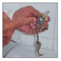
8 The main body of the assembly kit is fixed to washbasin assembly bolt, with the help of nuts, as shown on the above.
