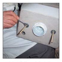
2 Install the flushing mechanisms to the cistern.
