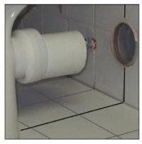
Slide the eccentrical trap adapter to the outlet of the wc pan. Calculate the gap , which is needed for extension for the waste piping.
