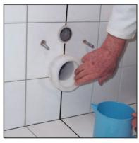
Prepare the waste outlet. Slide the eccentrical trap adapter in.
