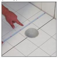
Set the distance between the outlet of the wc pan and the finished wall. Prepare the waste water outlet on the floor.
