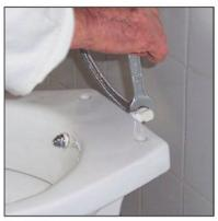
6 Connect hidden lustration pipe and connection adapter with 3/8" flexible pipe on WC Pan.
