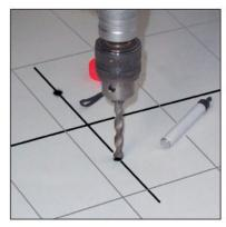
6 Drill the marked points with suitable drill bits and insert the raw plugs.
