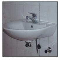
Drill the holes with suitable bits, insert raw plugs. Install the interval taps for clean water and washbasin tap. Slide the plastik bushes and washers, screw the nuts.
