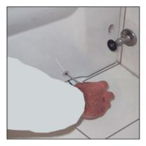
Slide assembly screws trough plastic bushes and screw to main mounts at both sides of the bidet.
