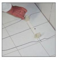
Join the markings at the 5th figure horizontally. Intersect it also with the vertical axis drawn before.
