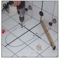
A Drill the marked points and insert the plugs.
