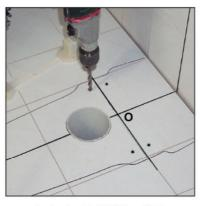
1 1 Overlap the strip's "+" sign with the intersection of axis on the floor. Now, mark the holes of the main mounts on the strip. Drill them.
