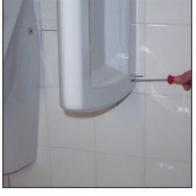
After fixing the wall seperator, its essential to apply silicone based paste troughoud the joinning edges of seperator and finished wall.
