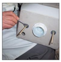
4 Install the flushing mechanisms to the cistern.
