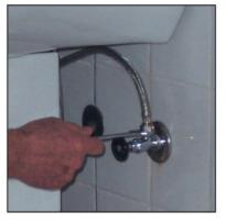
After fixing the washbasin, make the connections between interval taps and basin tap.
