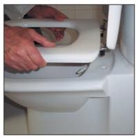
15 Each WC pan has its own seat cover, Thus, place the seat cover with its hinges on it, by sliding the screws trough installation holes on the pan.
