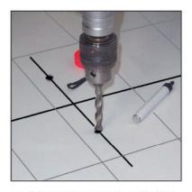
3 Drill the marked points with suitable drill bits and insert the raw plugs.
