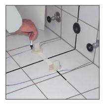
Join the markings at the 4th figure horizontally. Intersect it also with the vertical axis drawn before. Overlap the strip's "+" sign with the intersection of axis on the floor. Now, mark the holes of the main mounts on the strip.
