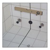
After installation of the carriage bracket; the waste water outlet and interval tap inlets are prepared and proceed on tile works.
