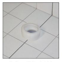
2 Place the eccentrical trap adapter to its location inside the waste water outlet.
