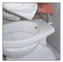
Connect hidden lustration pipe and connection adapter with 3/8" flexible pipe on WC Pan.
