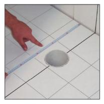
The gap between the waste water outlet and the finished wall must be set 250 mm. Draw an axis on the floor by using the mid-point of the waste water pipe.
