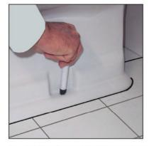
Keep this distance and mark the projection of the bidet and assembly holes on the finished floor.
