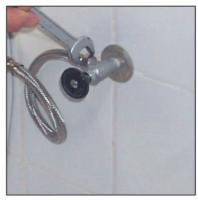
$\boldsymbol{6}$  Finish with the connections between interval taps and the bidet tap.
