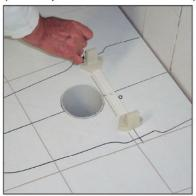
10 Join the markings at the 6th figure horizontally. Intersect it also with the vertical axis drawn before.
