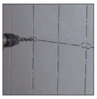
The front of the washbasin will be temporarily set to 800 mm. above the finished floor and the centres of assembly holes behind will be traced on the wall. Always use additional axis and centres to assist for a proper and balanced assembly process.
