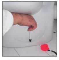
Bring the wc pan temporarly to assembly position. Mark the holes on both sides on to the finished floor.
